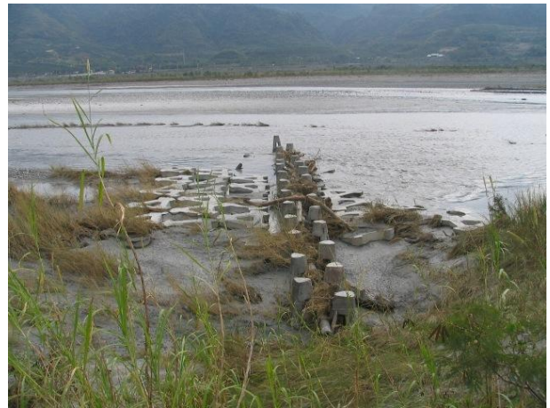
(13)玉里堤防丁壩掛淤營造棲地(93.08) (14)玉里堤防架樁丁壩縱向實景(93.12)
